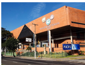
Fachada do MCT PUCRS Avenida Ipiranga, Porto Alegre/RS
