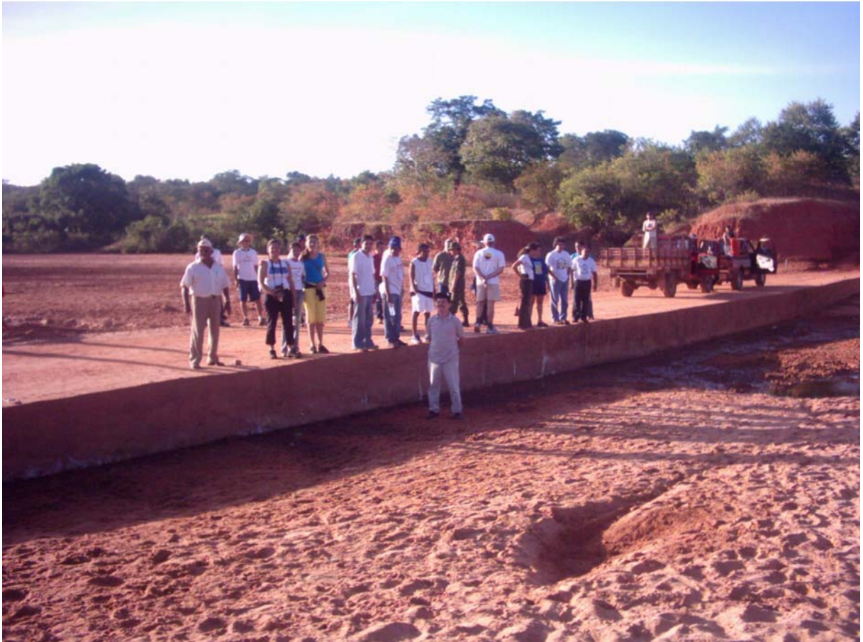
FIGURE 1.8 Boqueirão Bridge (80,0 m X 3,0 m X 3.724 m), over the Boqueirão River, in Gilbués, Piauí. (Photo: Luís Gonzaga, Ufpi, May, 2004.)
