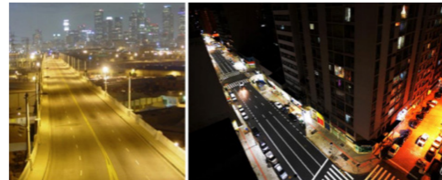
Figure 33: Comparison between zebra effect and uniform lighting
