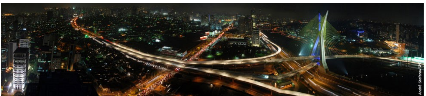
Bridge Octavio Frias de Oliveira (cable-stayed bridge)
