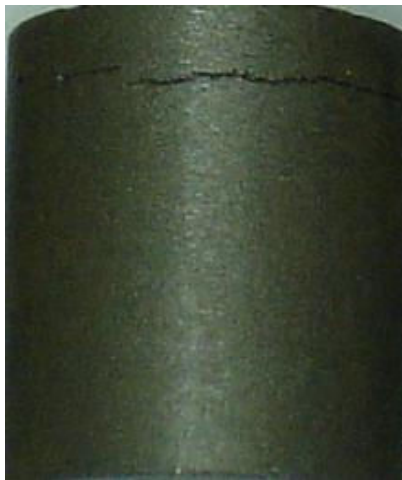
Figura 4 – Trinca transversal “OLIVEIRA (2010)”.
