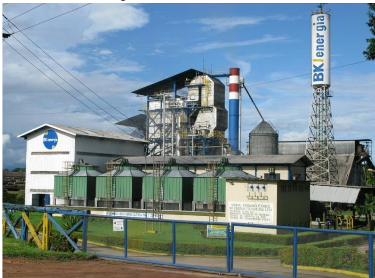
Figura 44. Usina BK Energia movida a biomassa florestal – Itacoatiara, AM.
