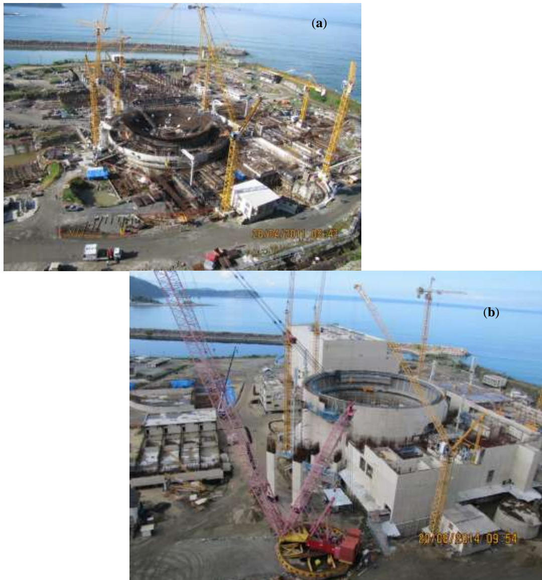
Figure D.1 - Angra-3 construction evolution - (a) 2011, (b) 2014
