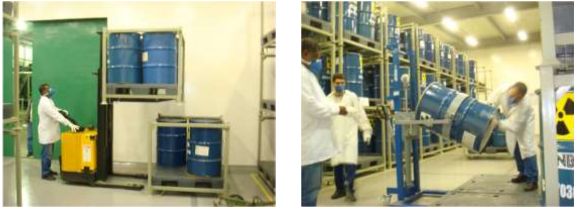
Figure D.2 – Low-level waste storage facility (DIRBA) at FCN
