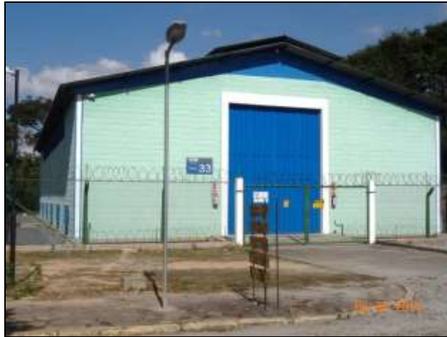
Figure H.3 – DFONTE - Intermediate Storage Facility Building -CDTN
