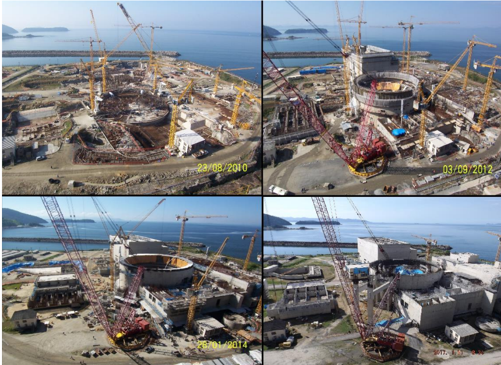
Figure D.1 - Angra-3 construction evolution – 2010/2017
