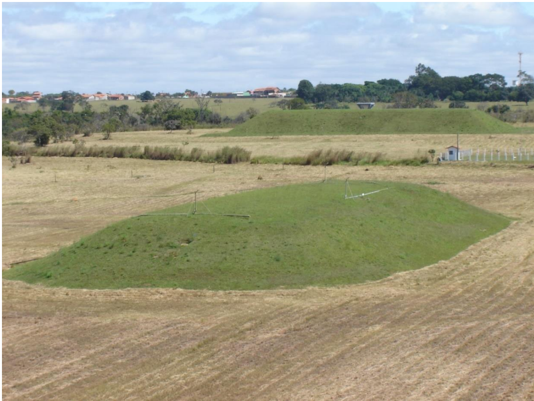
Figure D.3 - FRONT: Great Capacity Container; BACK: Repository at Abadia de Goiás
