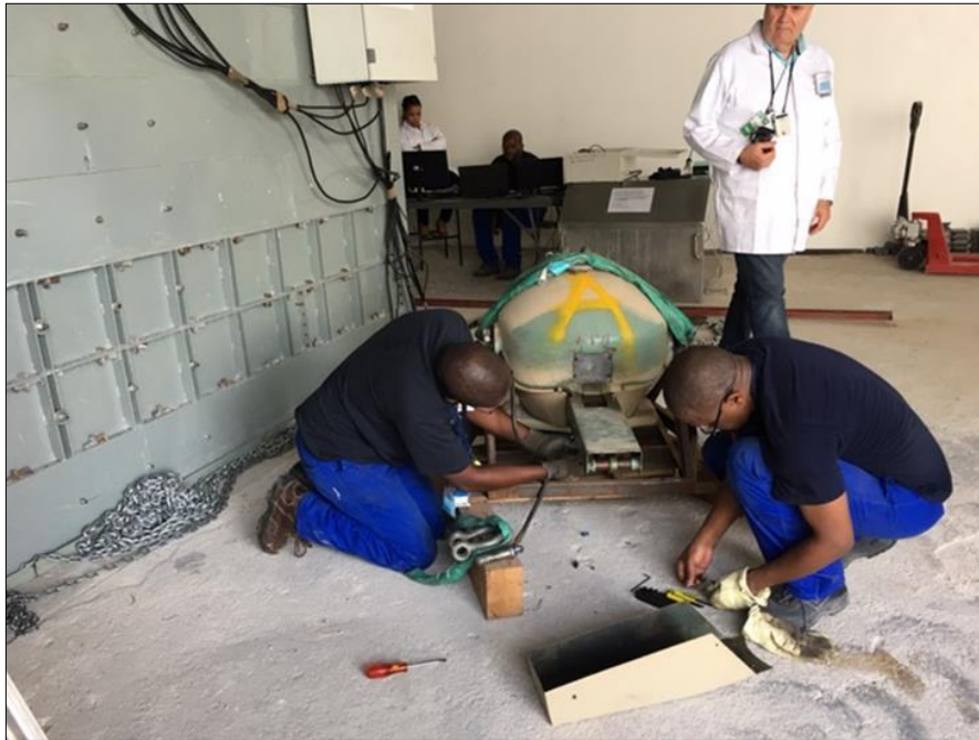
Figure I.1 – Teletherapy head pre-dismantling
