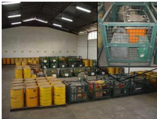
Figure 6.1: CNEN regional deposit in Brazil where radioactive material is stored in appropriate containers after collection from different sources. [66]
