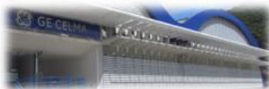
14Bis Building New Make & Overhaul
