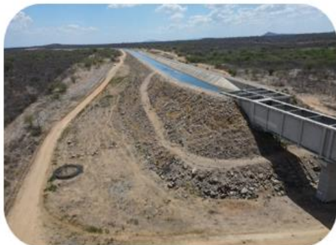
Segmento de Canal CN03 (WBS 1207) Roço - 219.460,84m 3
