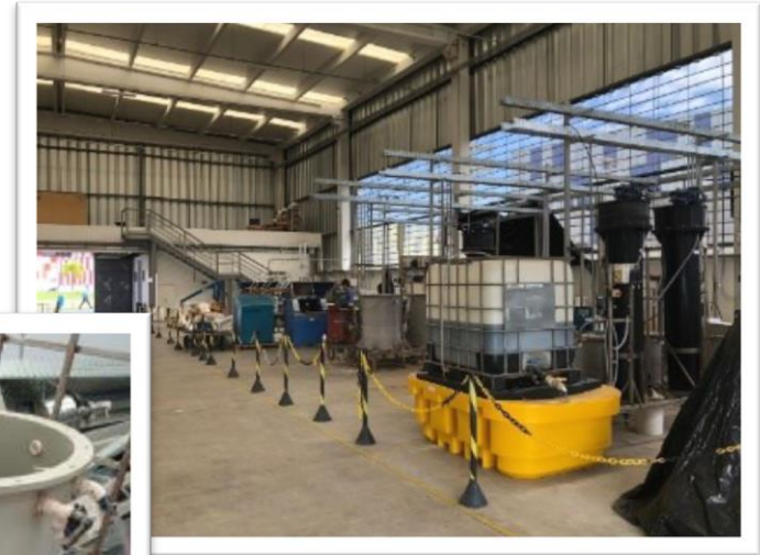
future pilot plant installations
